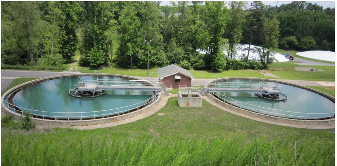
Water treatment site
